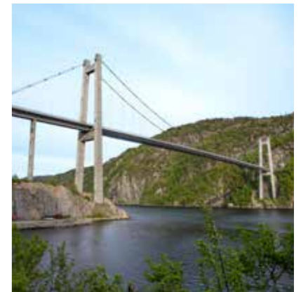
FEDAFJORD BRIDGE IS A SUSPENSION BRIDGE ACROSS FEDAFJORD IN KVINESDAL MUNICIPALITY. IT IS 566 M LONG WITH A MAIN SPAN OF 331 M AND A 50 M MAST CLEARANCE.
